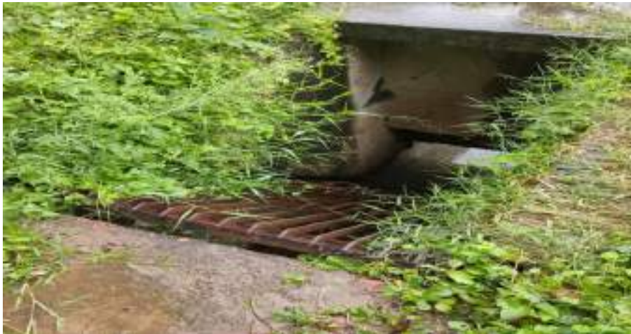
33 MLD STP at Mattagajpur Cuttack
