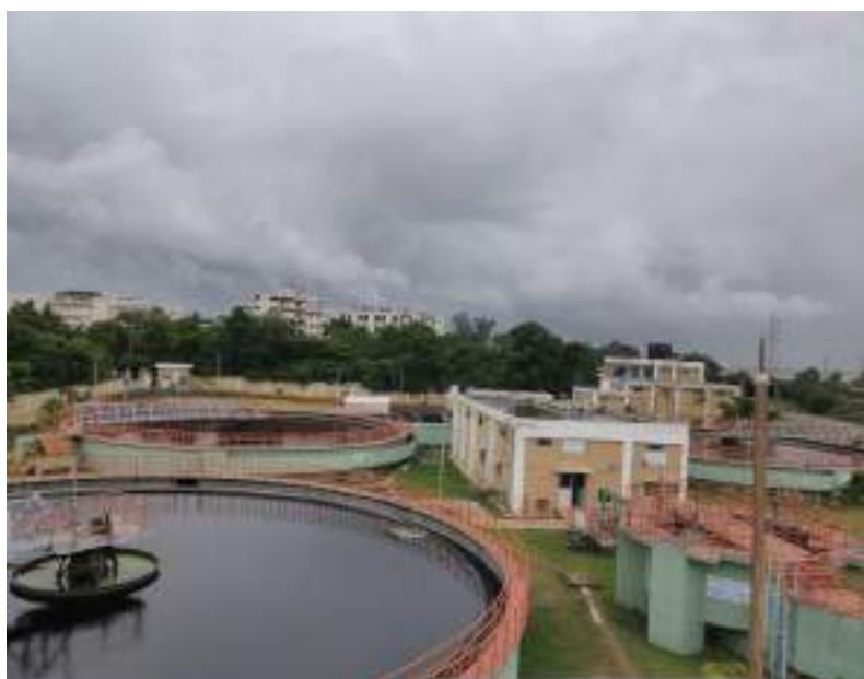
36 MLD STP at CDA-Bidanasi area of Cuttack
